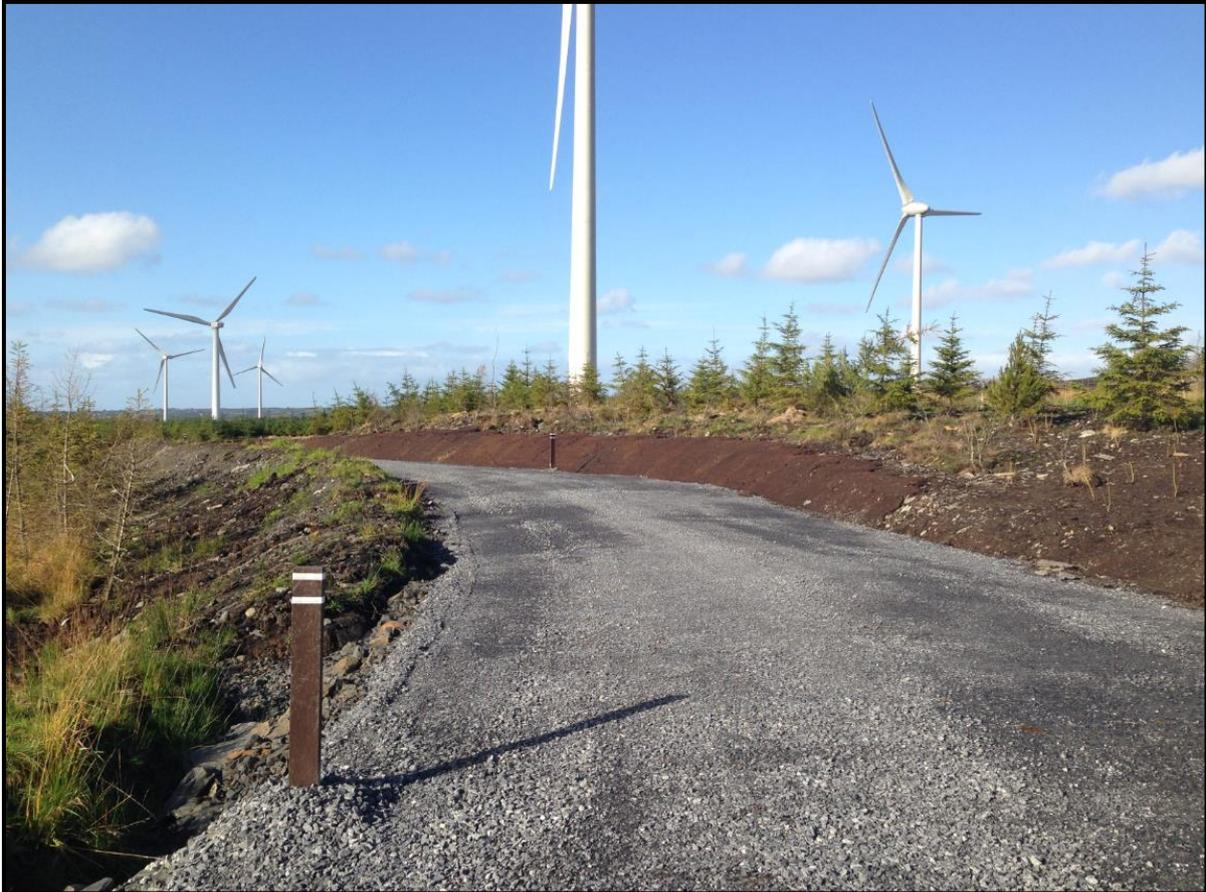
Figure 2 – Typical new excavated road on a wind farm
